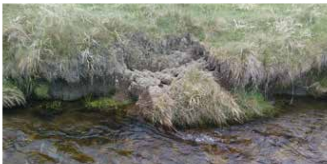
Streambank erosion is not always caused by livestock.
