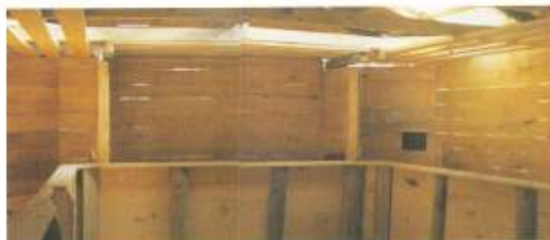
Horseshoe-shaped race, under construction
